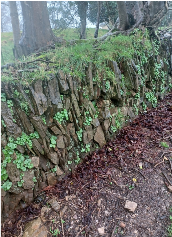
Towards point B and temporary diversion
